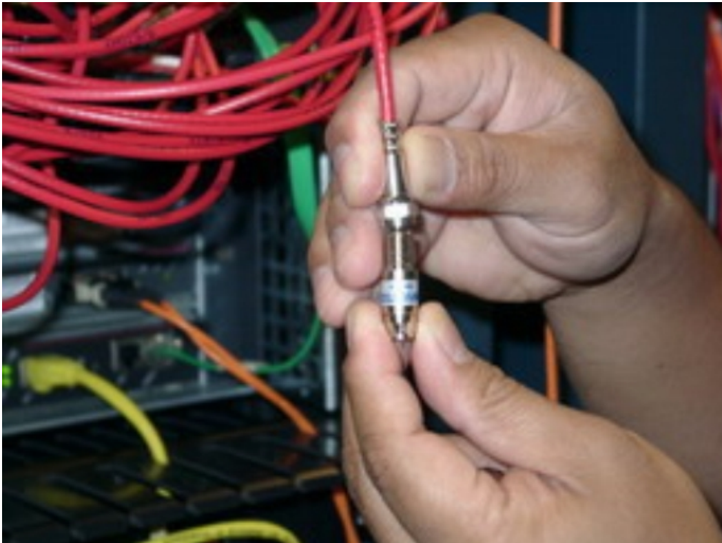
Figure 6: Adding the Attenuator to the Downstream Cable
